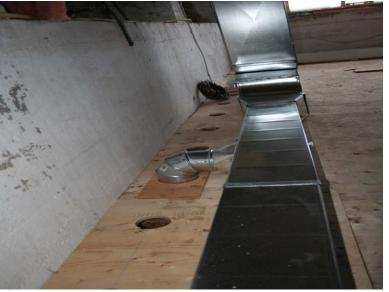
Air Gap Supply and Return Ducting
